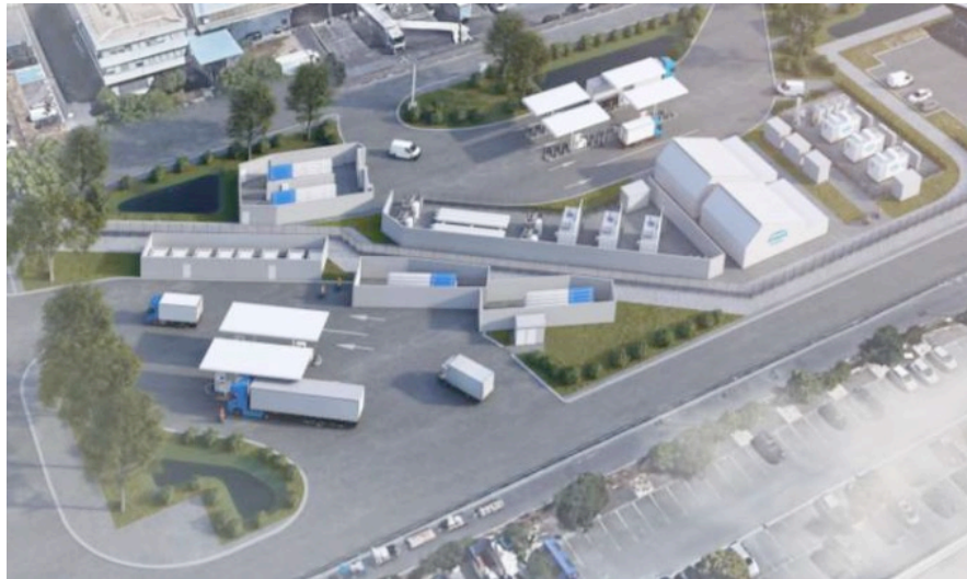
Figure 28 : GH2 and Natural Gas refuelling station in the freight area of Paris-CDG Airport – Feasibility study Source: Engie Solutions
