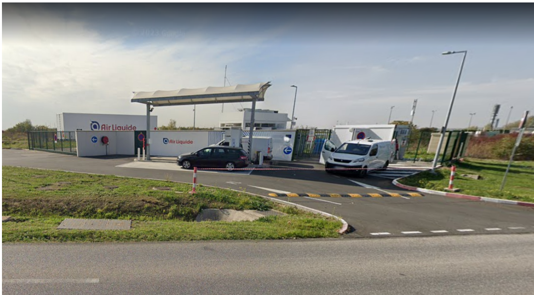
Figure 27 : H2 refuelling station for taxis at Paris-CDG Airport
