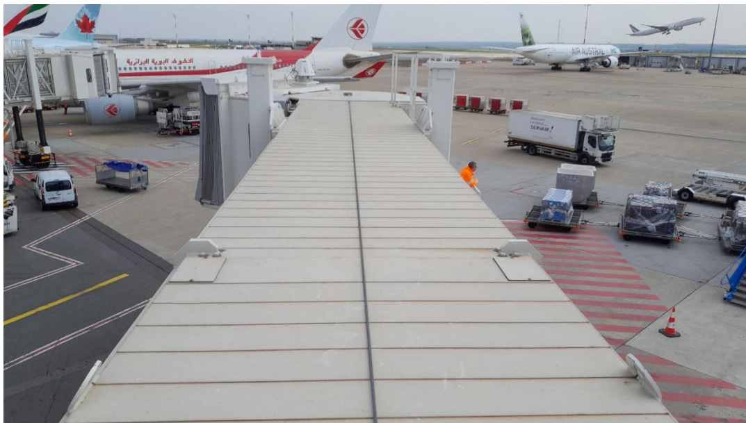
Figure 6: Example of a PBB roof
