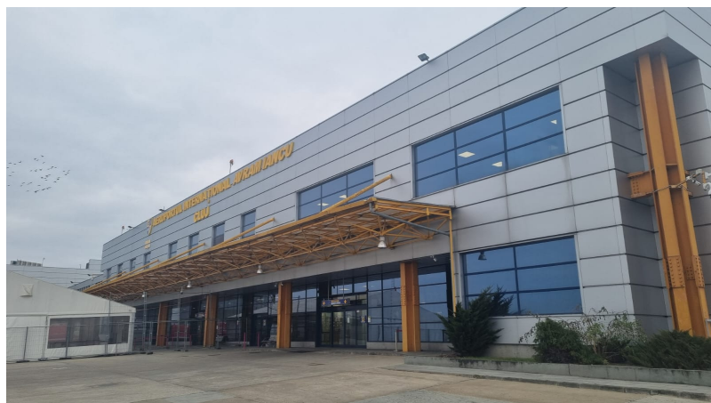
Photo. North façade
