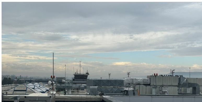
Photo. Non-circulating terrace floor
