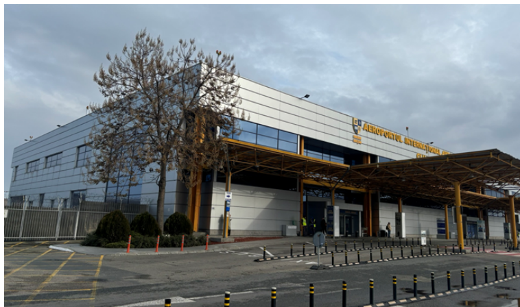
Photo. West and South façade
