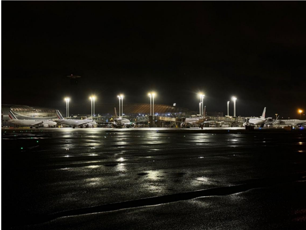
Figure 4: Final Terminal 2F LED apron lighting
