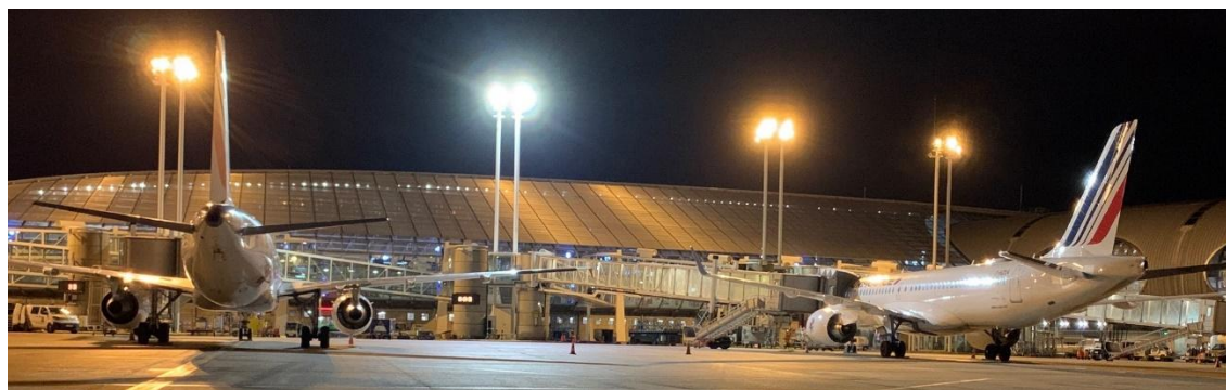
Figure 2: Terminal 2F first pole with LED fixtures
